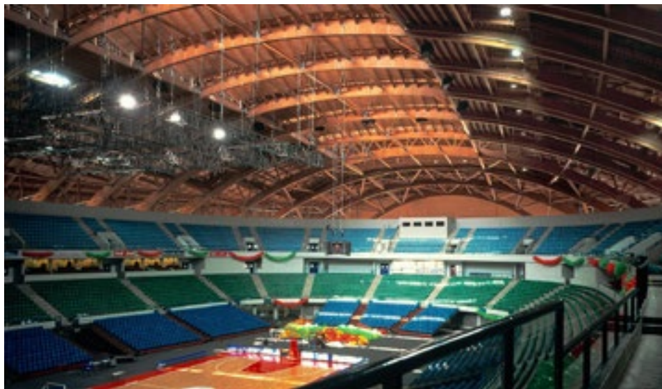
Wood Truss System
